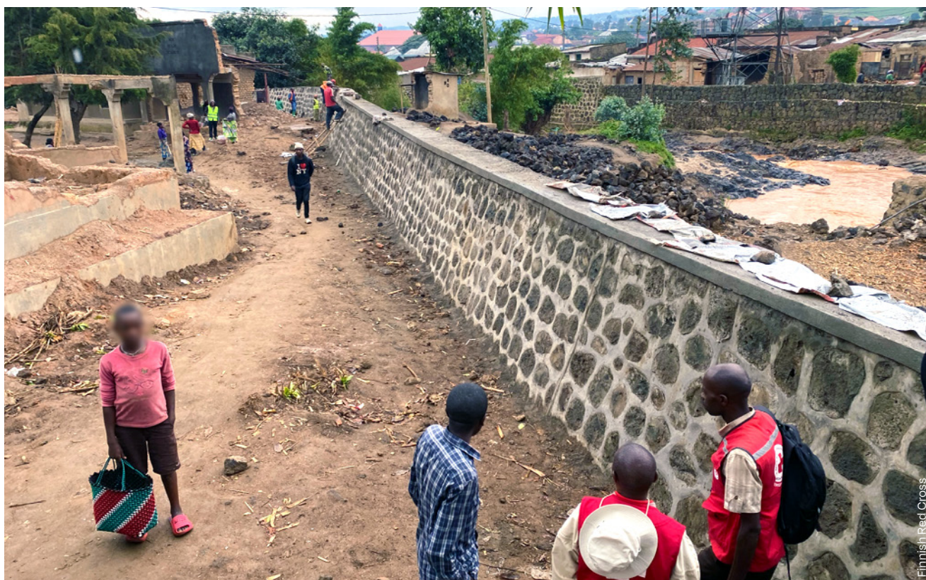
Flood retention wall was rebuilt after May 2023 floods in Mahoko cell, Kanama sector, Rwanda.
